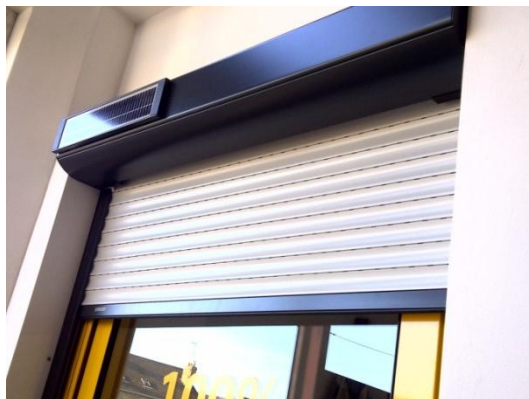
Fig. 9 ID 2 autonomous movable blinds operating with solar energy, 100% sun – 100 % independence [8]
