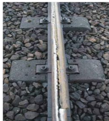
Cracking reaches surface
