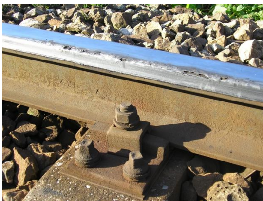
Fig.11 shelling on the rail
