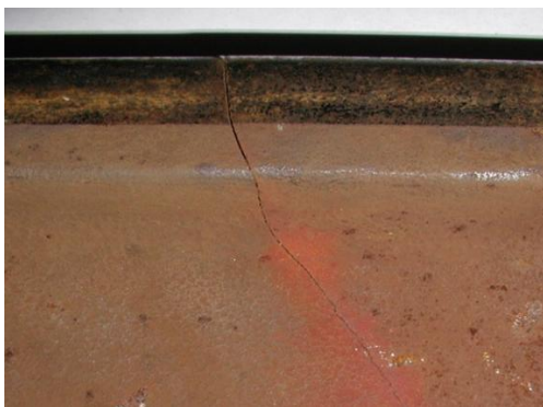
Fig. 1 transverse cracks
