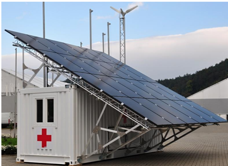
Fig. 2 Container dressing station with an island power plant based on renewable source of energy
